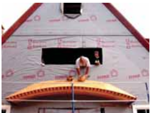
Placing crowns on our new construction
